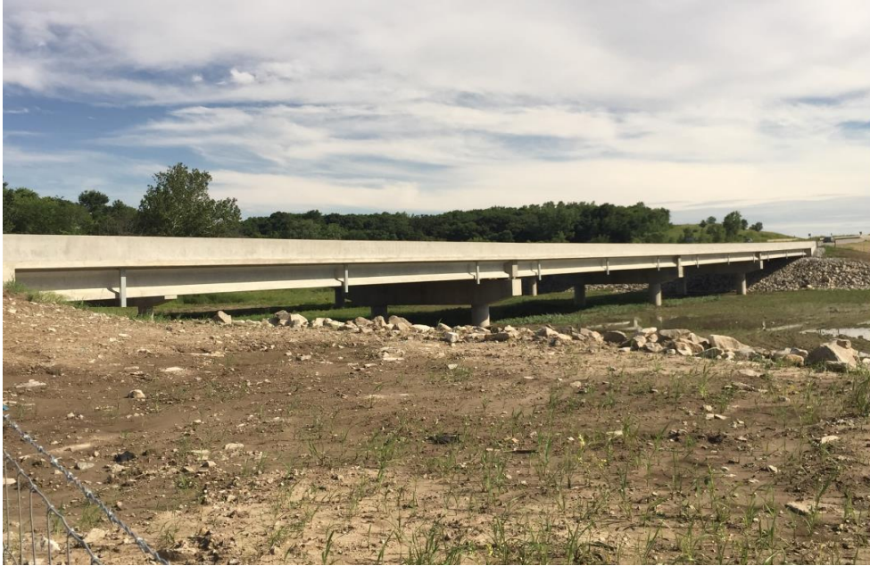
Fig.1: US 65 Des Moines River South Overflow Bridge
